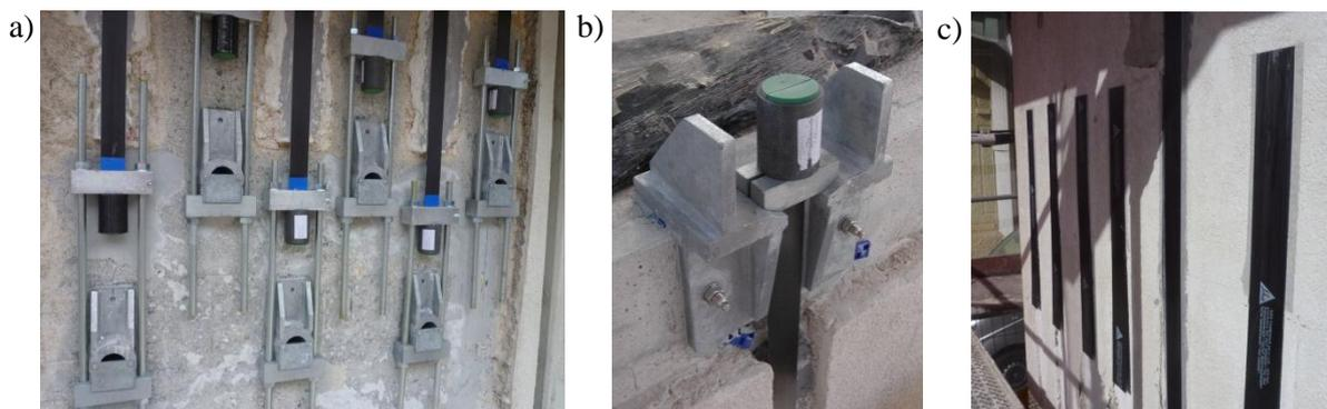
**Figure 6:** a) Movable anchor, b) Fixed anchor, c) Non-tensioned CFRP plate forming a displacement saddle
