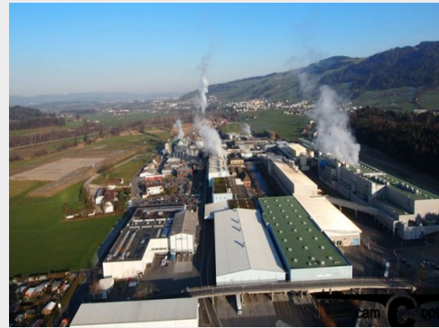
Beam strengthening Paper mill "Perlen", Switzerland
