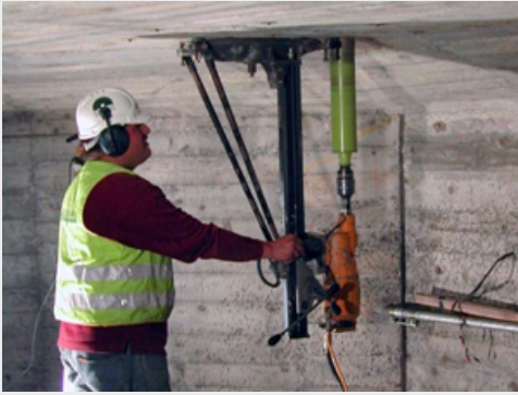
Step 1: Drilling for the anchors
