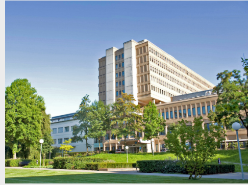
Earthquake strengthening Hospital Aarau, Switzerland
