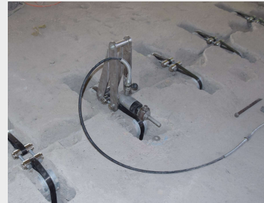
Tensioning process with clamping plier
